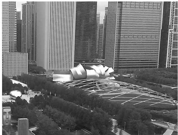
FIGURE 3: Jay Pritzker Pavilion, Millennium Park, Chicago, by Frank Gehry.
